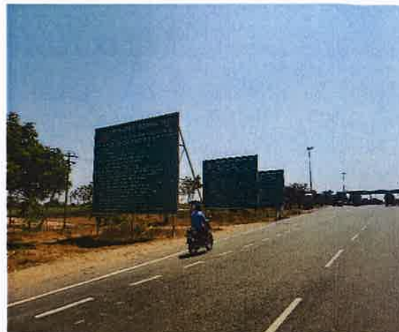
Pullur Toll Plaza
