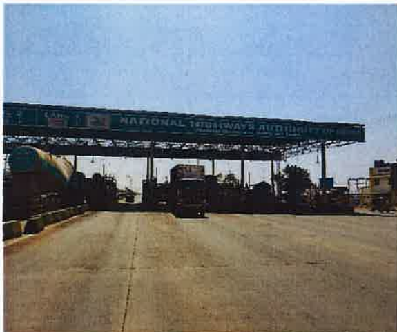
Pullur Toll Plaza
