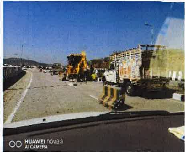
Repairing Work at Chittorgarh to Kota Stretch
